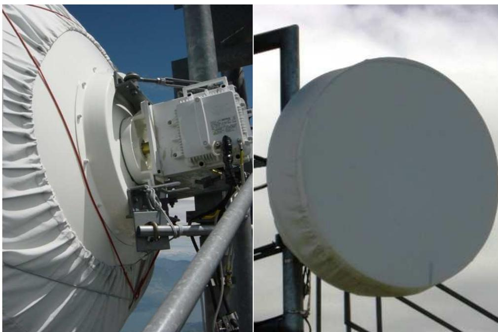
Figure 5 - Teflon cover from Stockhorn 16 months after installation
