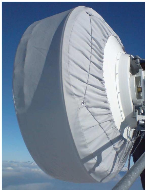
Figure 1 - Anti-icing Teflon cover
